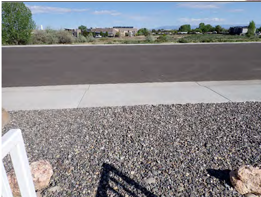
View across paved dam crest from walkway.
