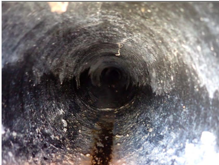
Internal view of filter collar drain outfall.
