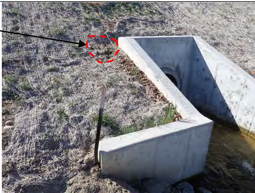
Right side of downstream outlet structure.
