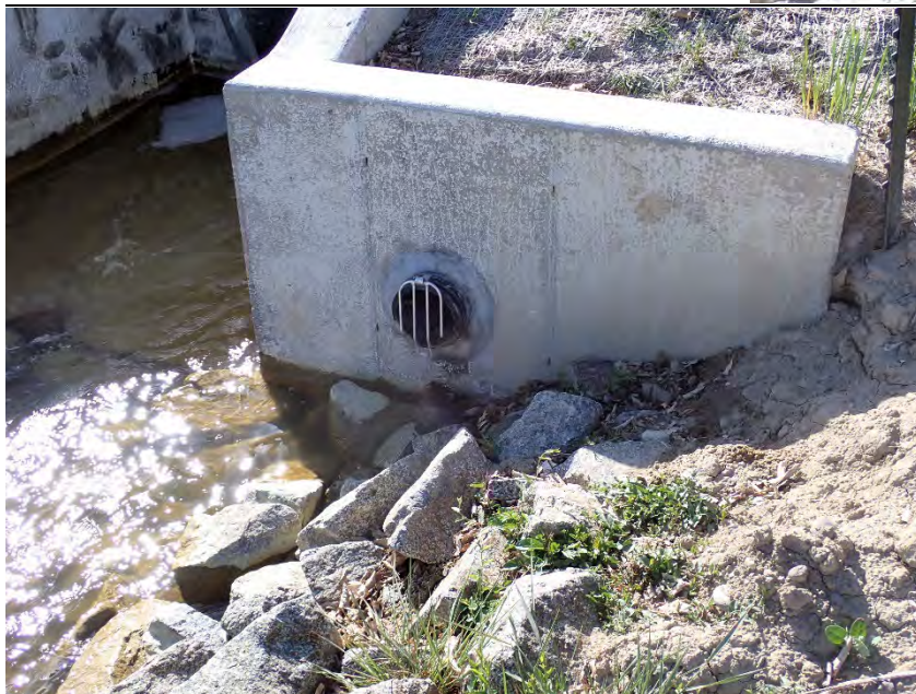
Close-up of filter collar drain outfall. Slow drip flow observed during inspection.
