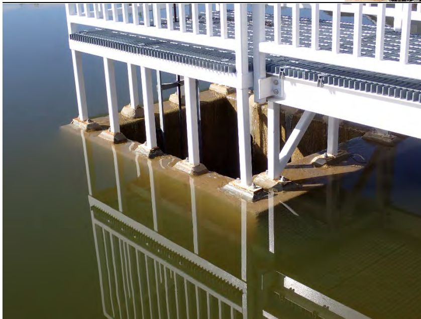
Right side of trashrack bars and combined service/emergency spillway drop structure.
