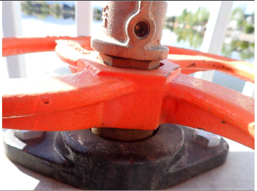
Stop nut flush with gate stem at full closure appears correctly set.
