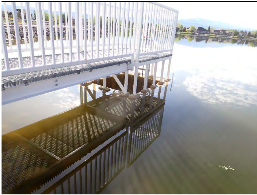
Left side of trashrack bars and combined service/emergency spillway drop structure.
