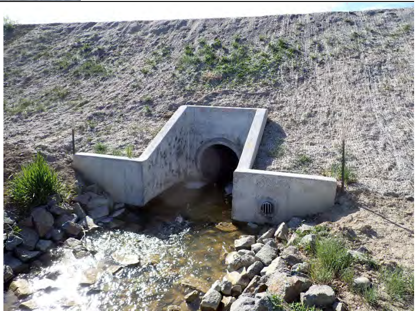
Downstream outlet structure.
