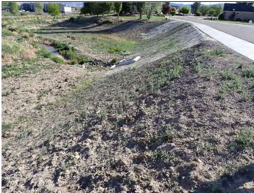
Downstream slope from left abutment.
