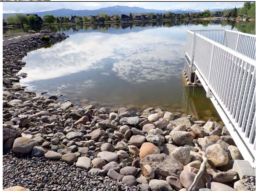
Upstream slope and right side of outlet gate access walkway.
